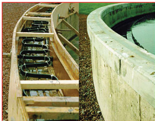
Final Settlement Tank de-icing
