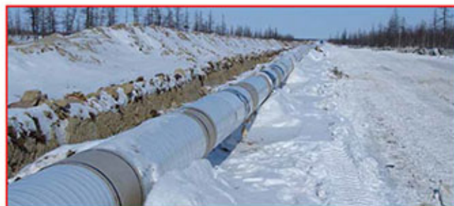
Completed Skin Trace system prior to burying
