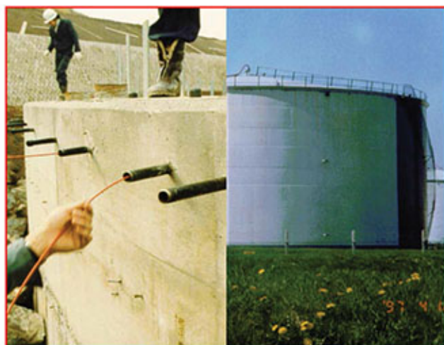
Tank base heating
